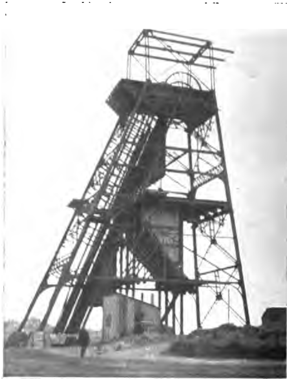
Fig. 3. Steel Head Frame, G. Pabst Iron Mine, Oliver Iron Mining Co., Ironwood, Mich.
